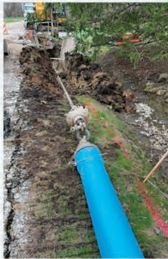
Watermain Installation via Horizontal Directional Drilling
