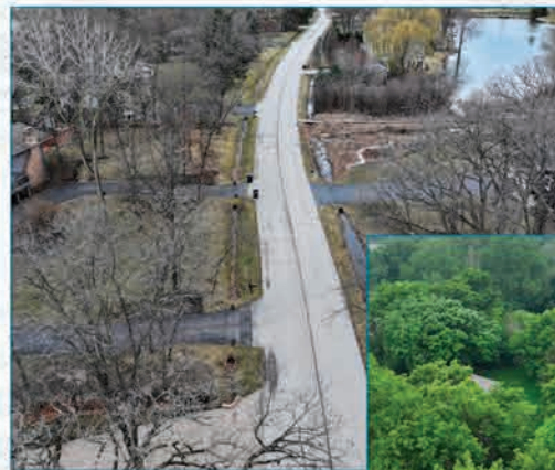
Cranbrook Road Before Roadway Construction
