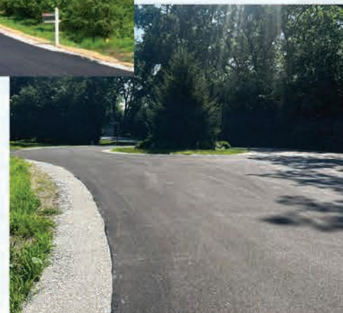
Cranbrook Road After Roadway Construction
