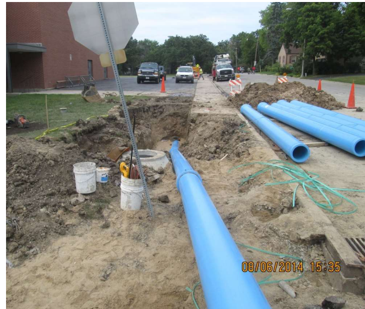
Horizontal Directional Drilled
