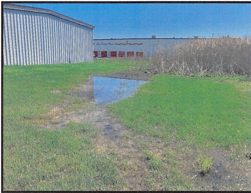
View of Wetland A – facing NE at south of building, inundated
