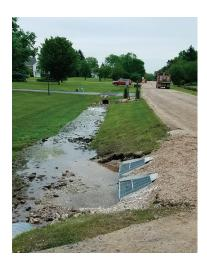
Cross-road culvert replacement, curb repairs & structure adjustments
